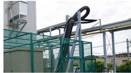
Figure 7. Bending parts of tri-axial superconducting cable (90 degrees, bending radius 1.5 meters)
