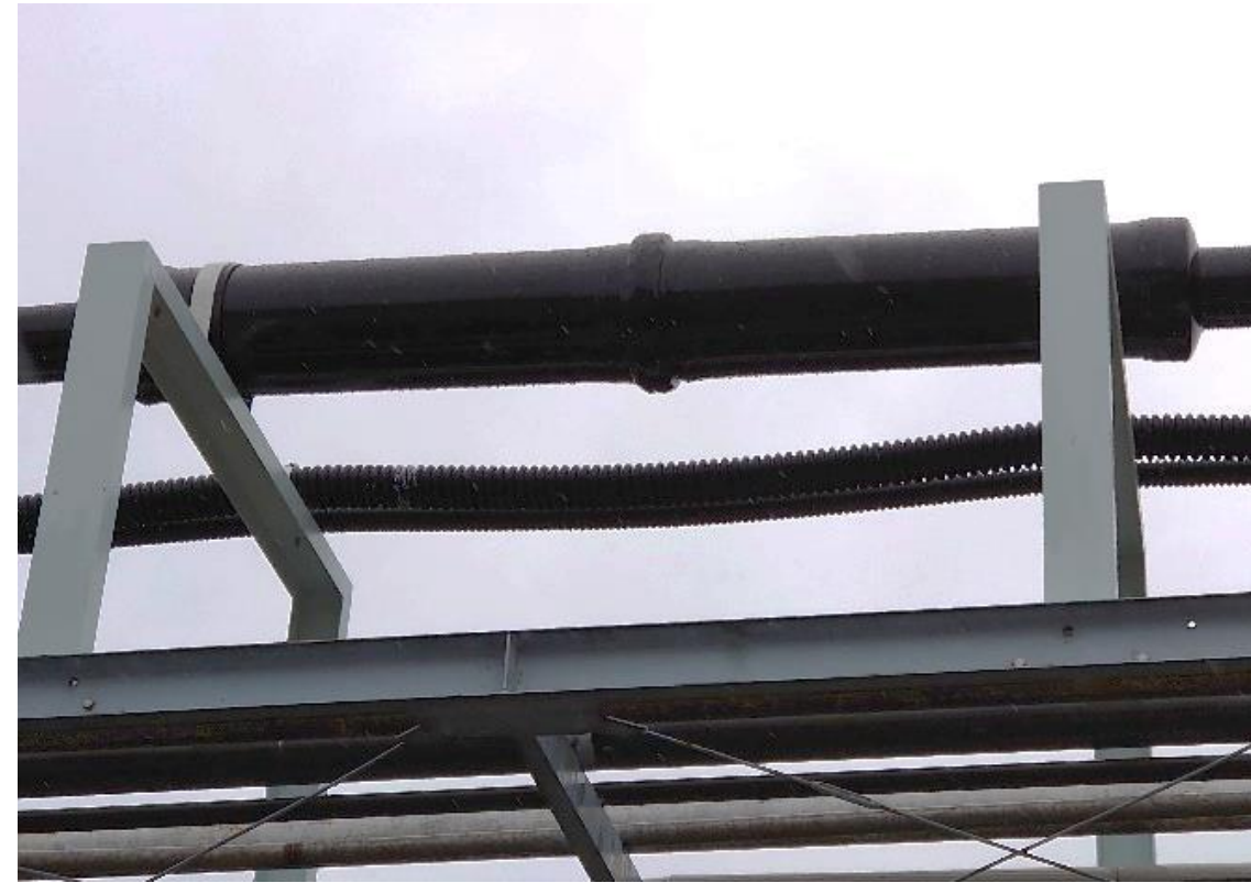
Cable joint Installation situation
