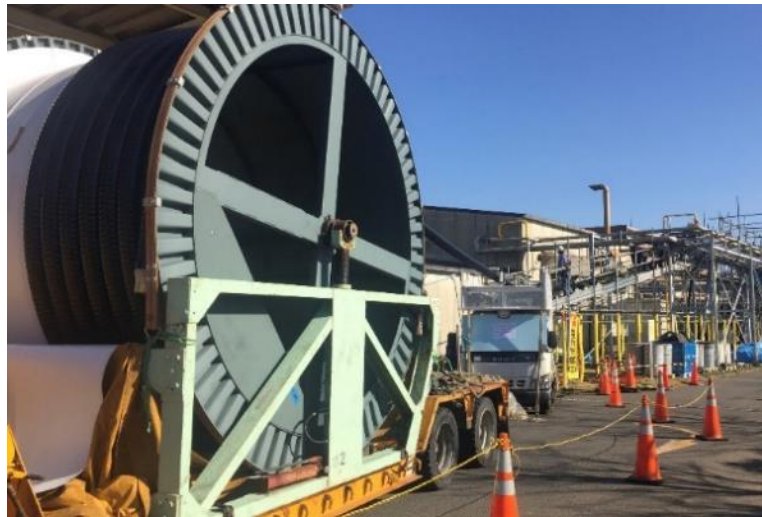
Before cable laying
