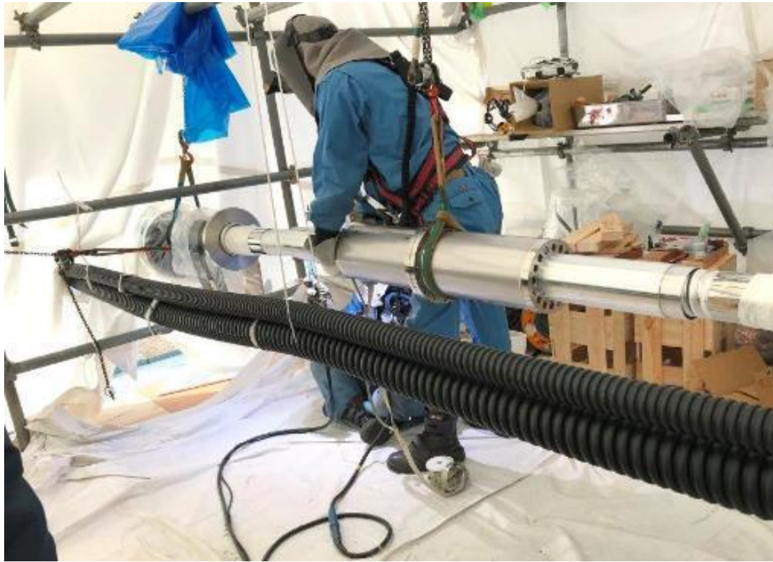
Cable joint assembly situation
