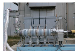
Terminal for triaxial superconducting cables
