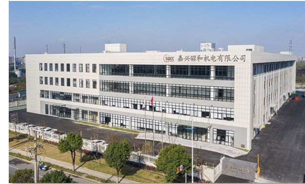
Wire harnesses China Jiaxing Plant
