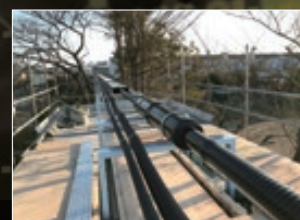
Three-phase coaxial superconducting cable system
