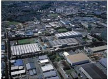
Sagami Office (Sagami City, Kanagawa Prefecture)
