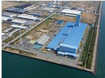
Aichi Plant (Toyokawa City, Aichi Prefecture)
