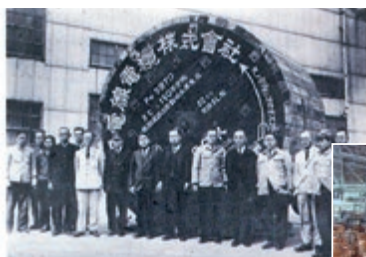
Shipment of high-voltage cables (Photographed in 1939)
