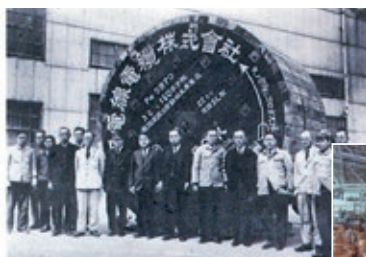
Shipment of high-voltage cables (Photographed in 1939)
