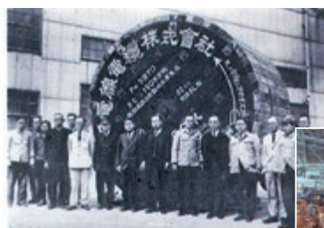
Shipment of high-voltage cables (Photographed in 1939)
