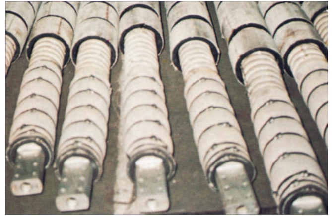
Covering in the installed condition
