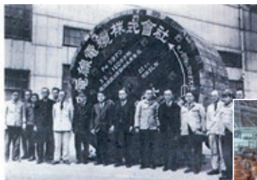
Shipment of high-voltage cables (Photographed in 1939)
